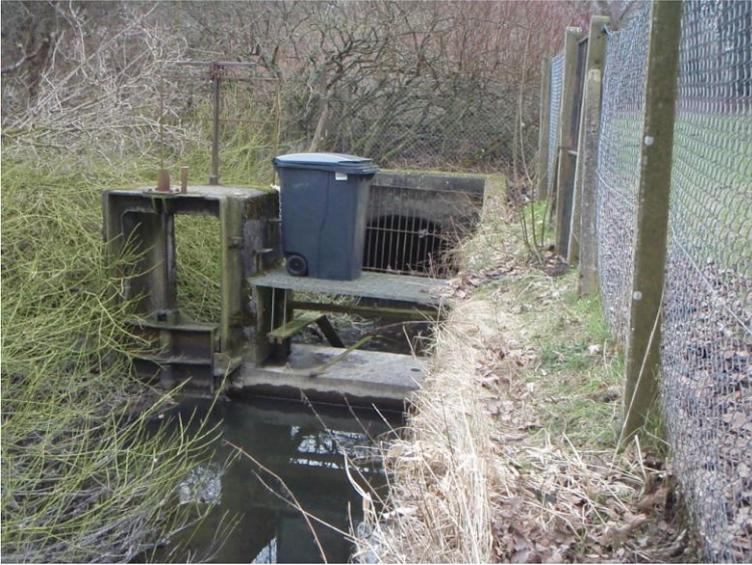
Of the three, the bar screen appears to be the structure which is restricting discharge from the Loch. Some attempt is made to clear the screen and there are heaps of weed on the banking. The grade of weed looks fairly consistent, with only a few larger sticks.
