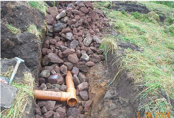
5031 is the distribution trench in the grass barrier strip. This was a sort of slow release mechanism which allowed the water trapped in the bund to trickle down to the burn.
