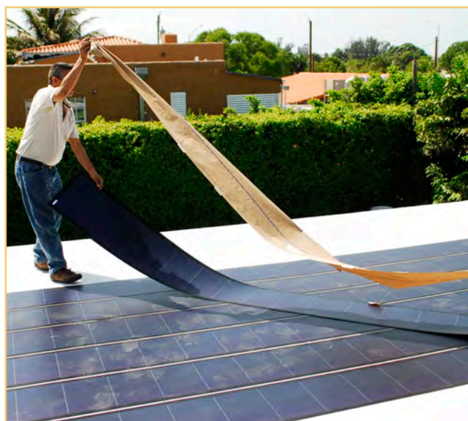
Thin film photovoltaic panels being installed onto a roof
