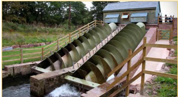
"Archimedes Screw" turbines
