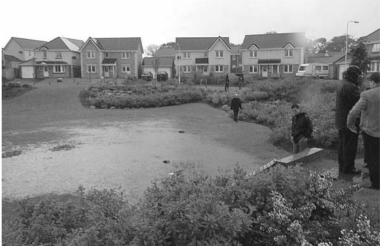
Stormwater filling an unlined SUDS detention basin. The clay content of the subsoil acts as a natural seal holding the stormwater and releasing it slowly. As in many soils in lowland Scotland, infiltration is not a major factor in SUDS planning.
