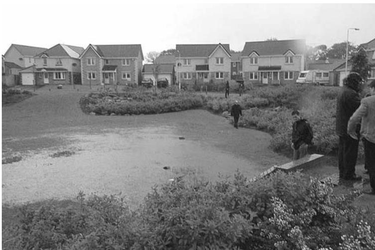
**Stormwater filling an unlined SUDS detention basin. The clay content of the subsoil acts as a natural seal holding the stormwater and releasing it slowly. As in many soils in lowland Scotland, infiltration is not a major factor in SUDS planning.**
