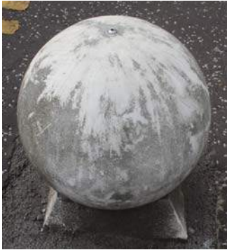
Large, cylindrical concrete bollards around West Port are a potential trip hazard and contrast with black cast-iron street furniture located elsewhere along the High Street.
