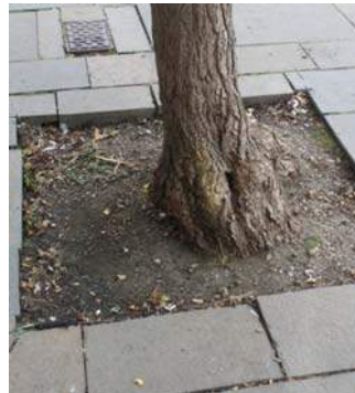
Right: Example of absence of tree grille in hard landscape and lack of underground support for tree.
