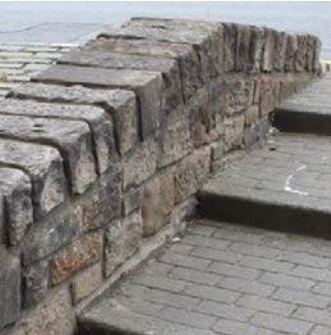
High quality existing stone materials could be reused to resolve levels issues.
