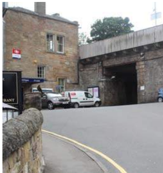
Entrance to station dominated by car parking and vehicular movement. Uninviting underpass leading to Station Road with no sense of what lies beyond.
