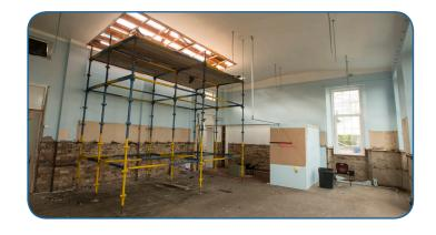
access improvements and on a series of small repairs and alterations to the existing roofs. While this is ongoing, all the necessary preparations are being made for the arrival of new mechanical and electrical systems as well as new internal finishes and some minor alterations to the layout of the existing building.
