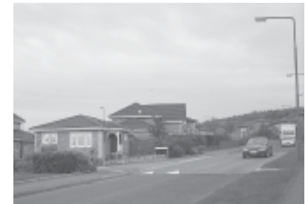
Raised junction, Livingston
