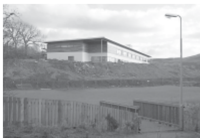
School under construction
