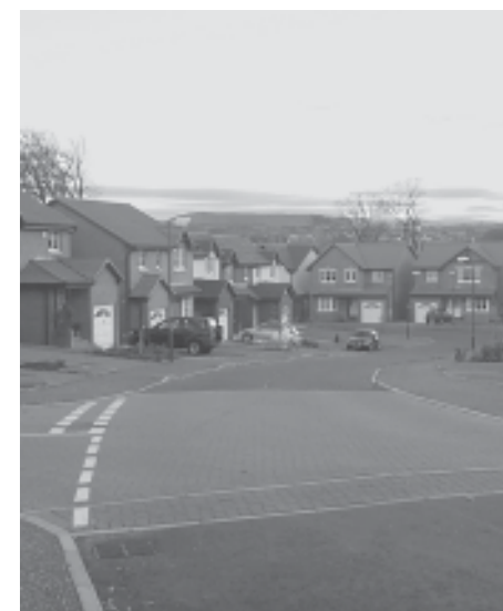
Top left: Parking court Bottom right: Lay by visitor parking
